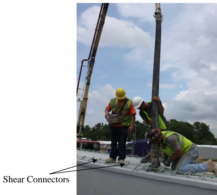
Figure 3-8 Placement of SCC, B0410 in Chesapeake, Virginia
