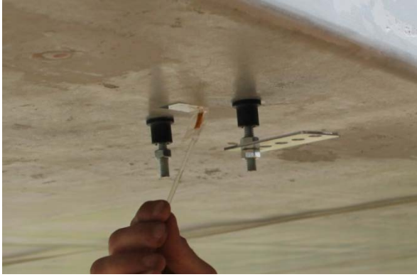
Figure 3-16 FRP Strain Gauge Placement, M-Bond Adhesive
