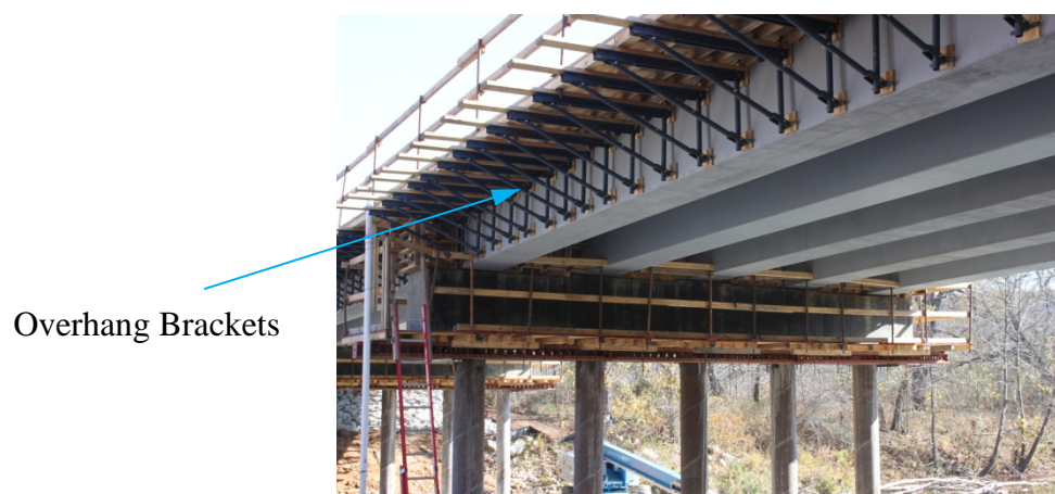
Figure 3-4 Construction of B0439 Superstructure
