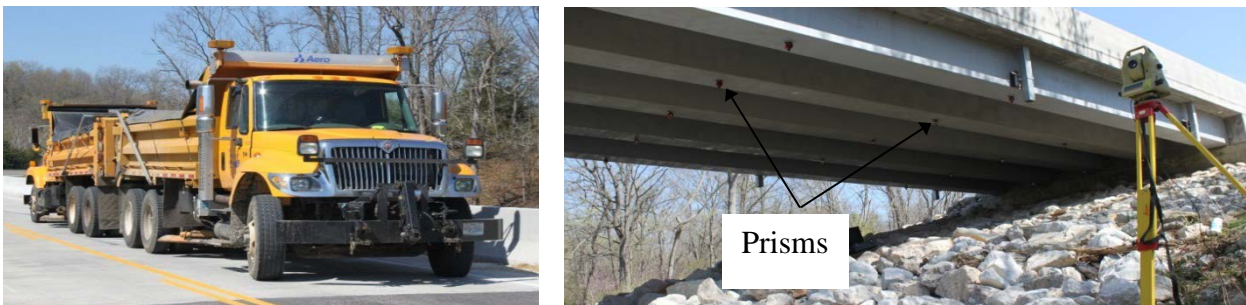
Figure 5-1 Load Test of Bridge B0439; MoDOT Trucks (Left Image); Total station and prisms (Right Image)
