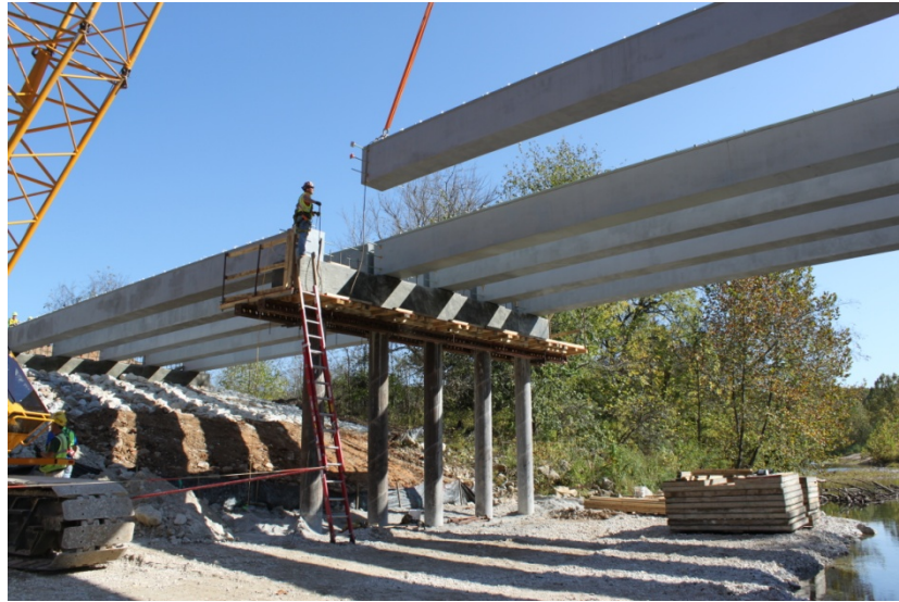
Figure 3-3 Installation of B0439 HCBs on the piers
