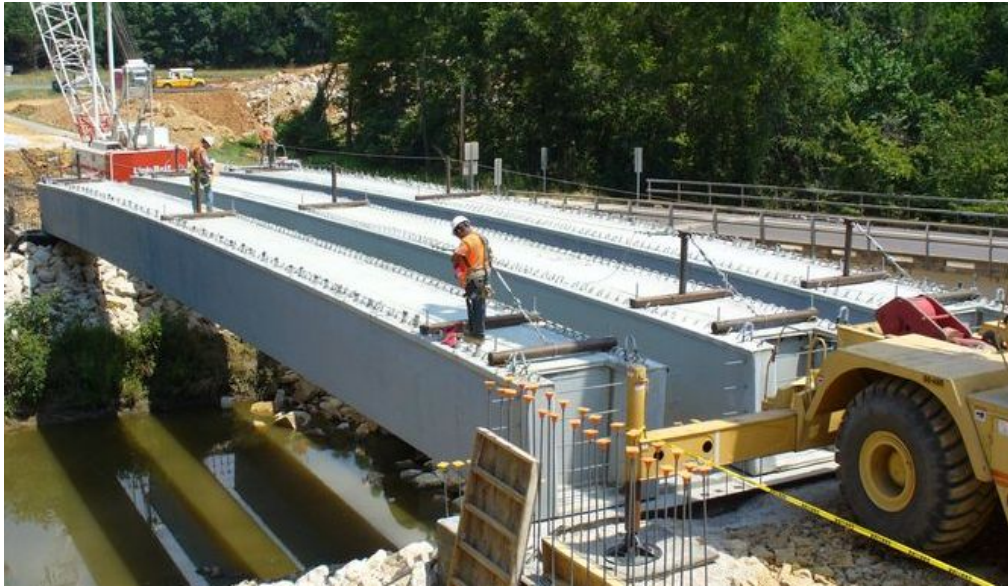
Figure 3-10 Erection of B0410 Double-Web HCBs
