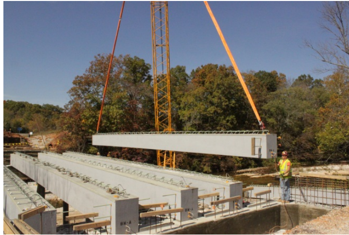
Figure 2-6 Erection Process of B0439 HCB
